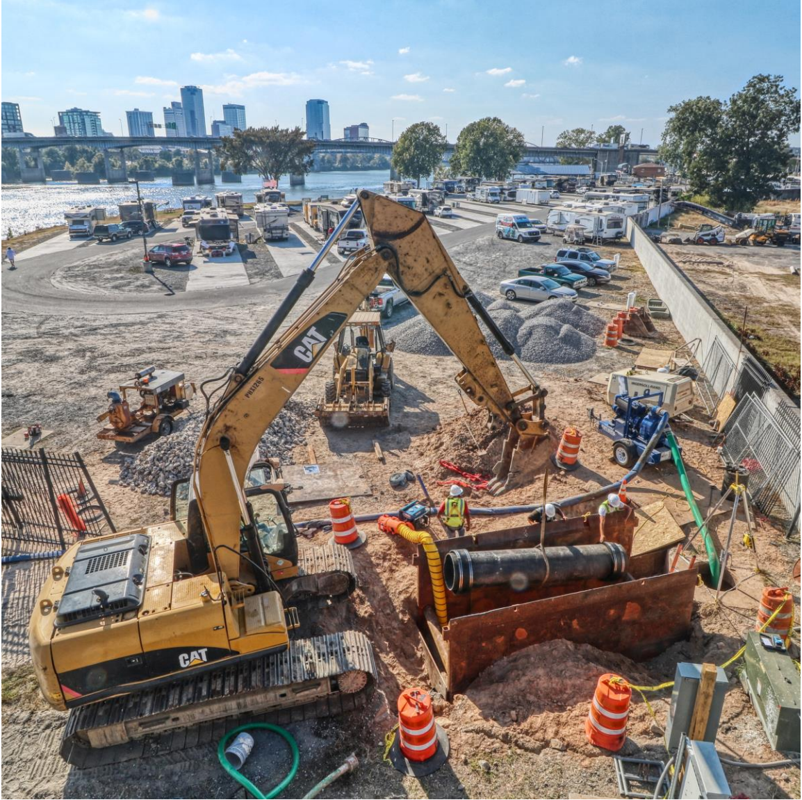
Point Repair on 24" Pipe near Arkansas River – July 2015
