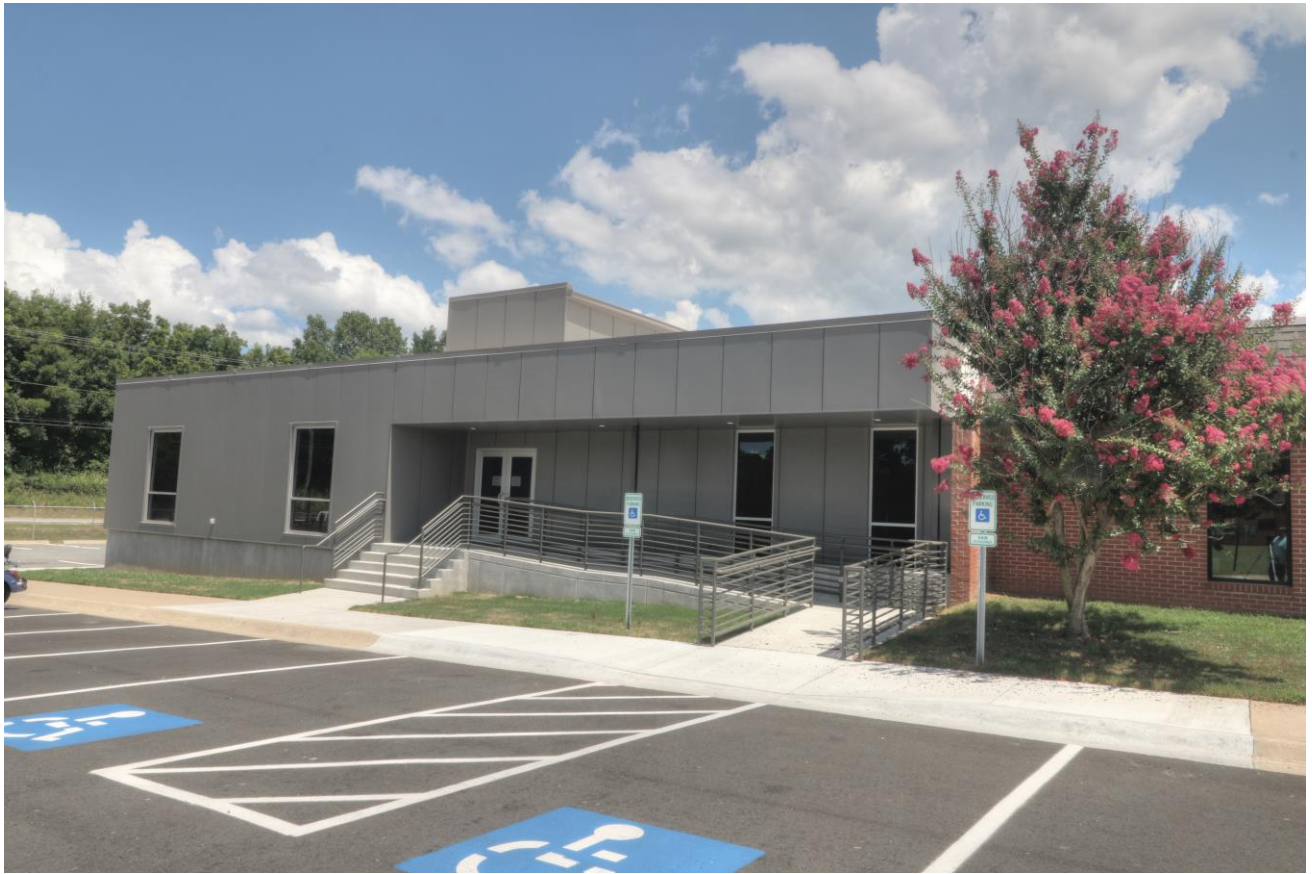
Collection System Building – August 2020
