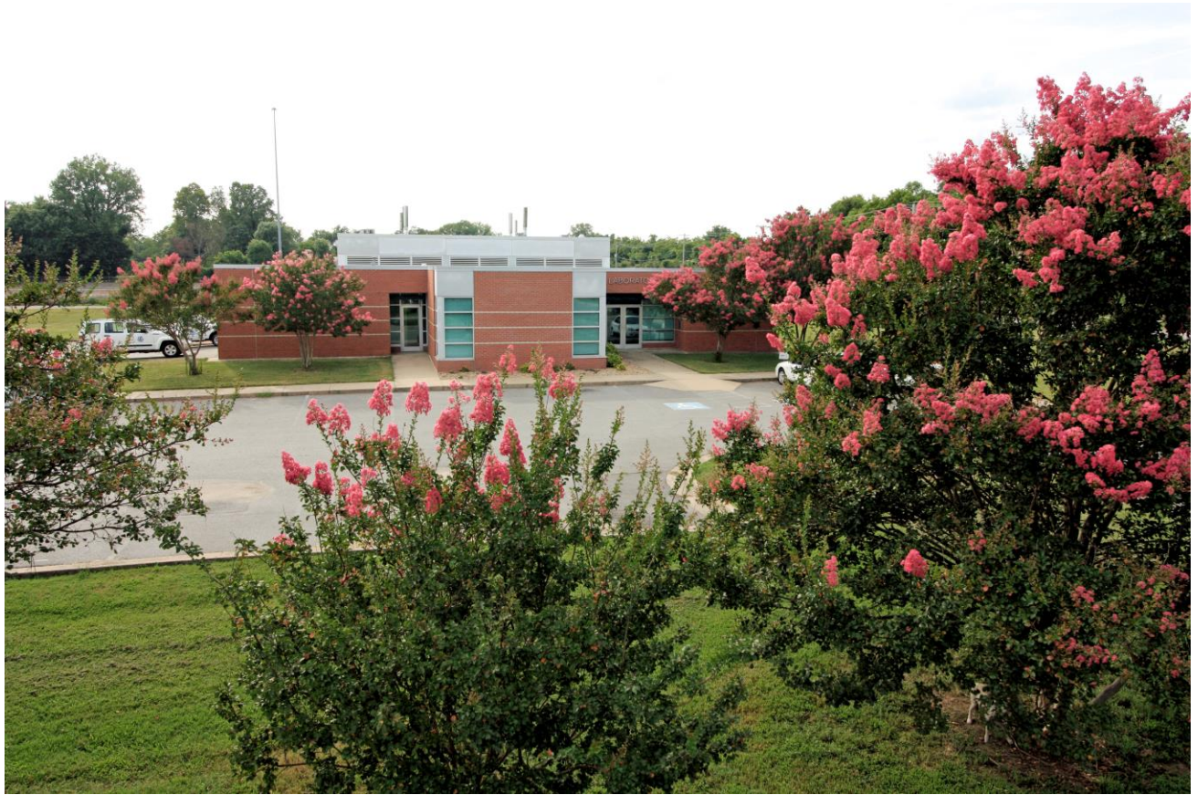
Laboratory Building at NLRW Faulkner Lake WRF – July 2015
