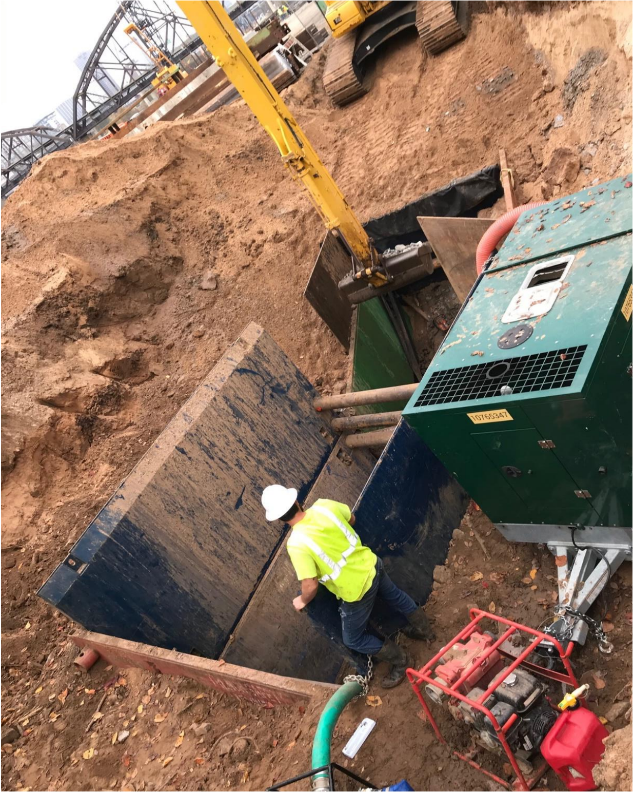
Upper Riverside Interceptor CIPP – November 9, 2020
