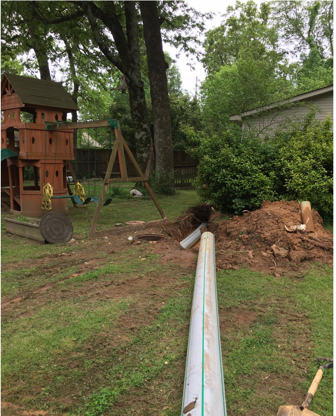
South Levy Pipe Bursting – September 18, 2019
