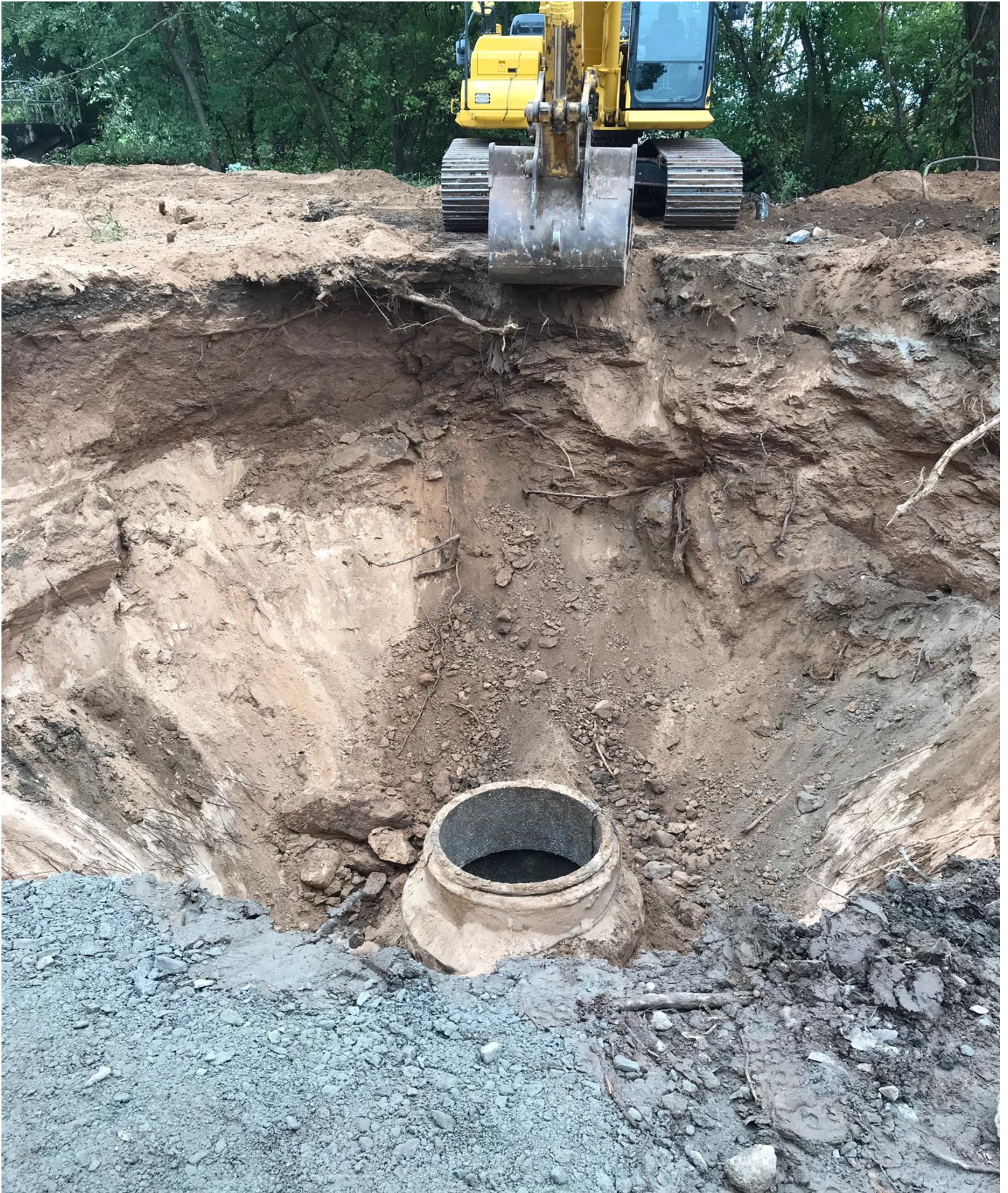
Upper Riverside Interceptor CIPP – November 6, 2020
