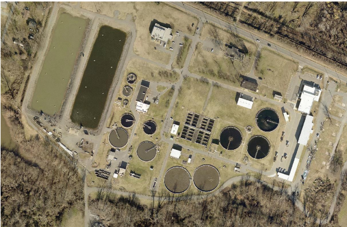
Faulkner Lake WW Treatment Plant
