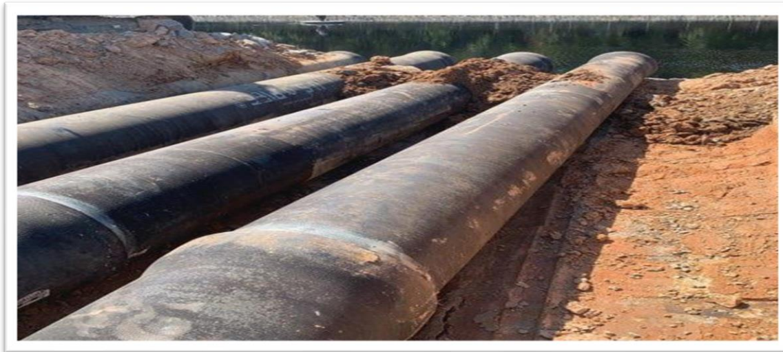
Faulkner Lake Piping Modifications
